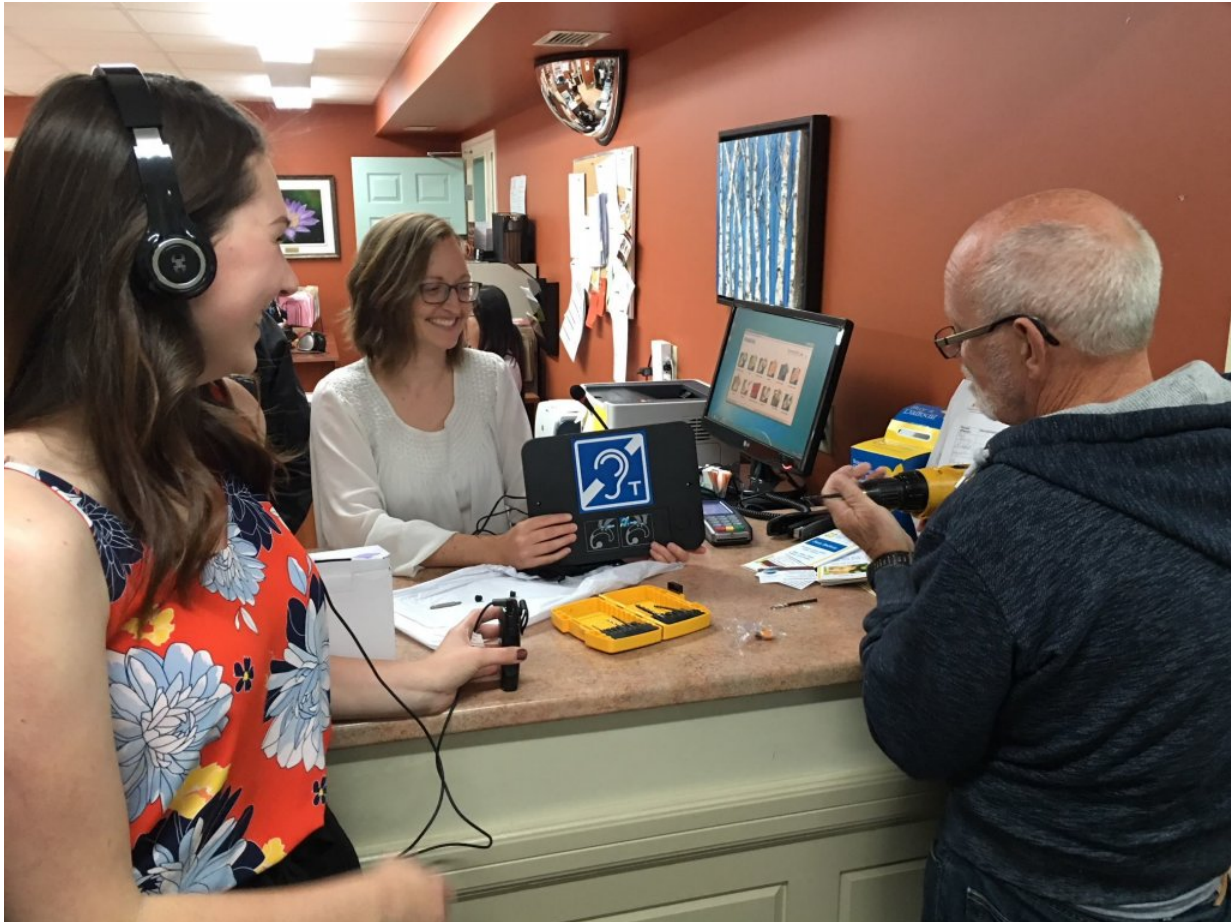
Jill Lowther, Taylor Burt, and Lee Ramsdell installing a counter loop at the town hall service desk.
