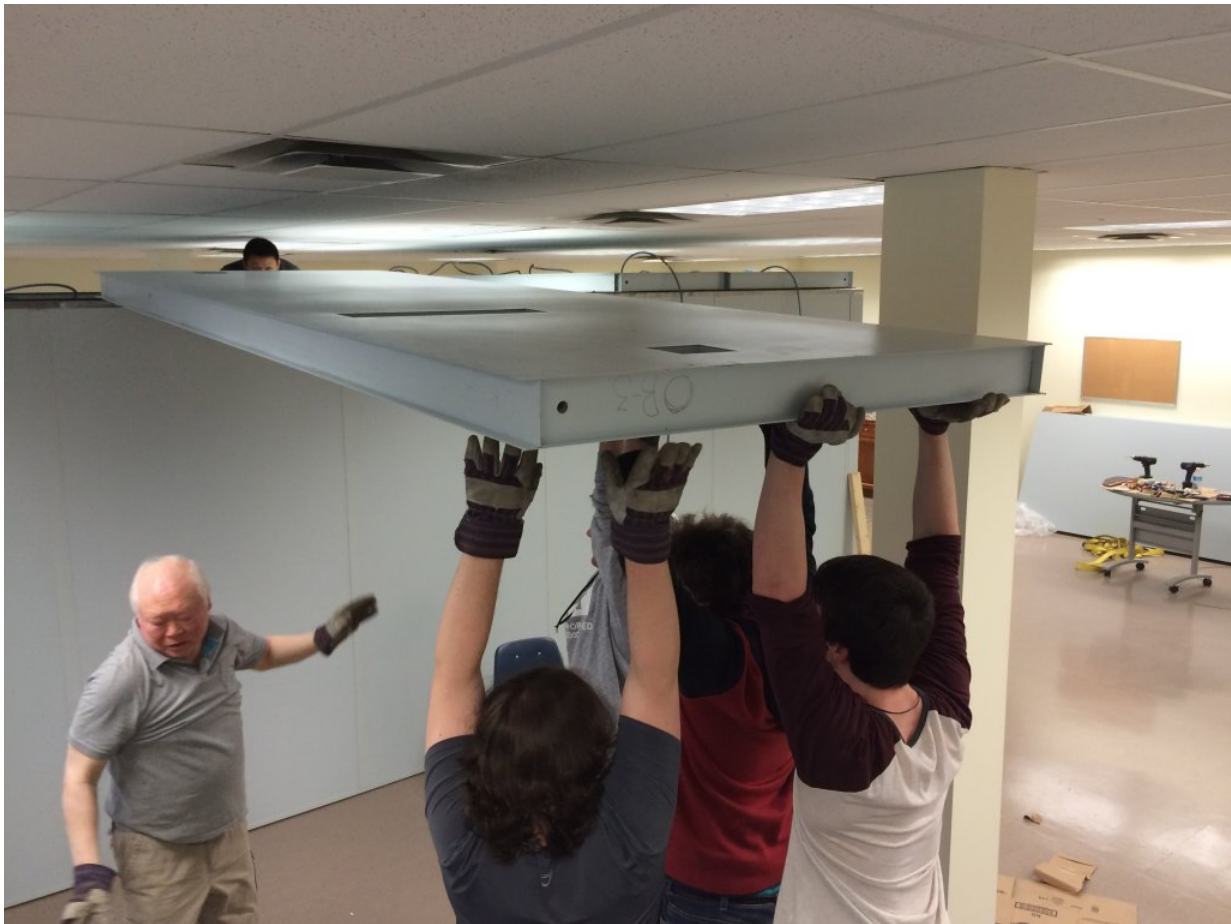
Assembling the booth.
