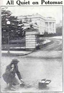
K. P. ROYCE of the Scientific Division of the Graybar Electric Company, making a test with the audiometer, at the East Gate of the White House. The noise measurement here was 25 units, showing that President Coolidge works comparatively free from interference.
